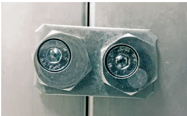
Figure 21: Connect inside type clamps with special eccentric M8x25 screws. Screws are included as separate delivery.
