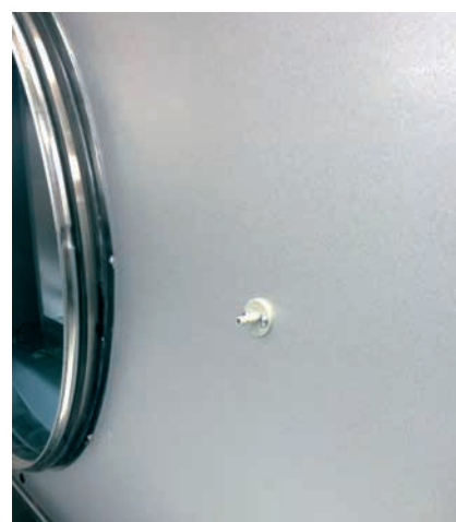
Figure 51: Tube connector for measuring duct pressure. User has to connect the attached tube to connector. The other end has to be connected to outlet air duct. The same procedure is required on inlet side. Inside CompAir, tubes must be connected to inside connectors.
