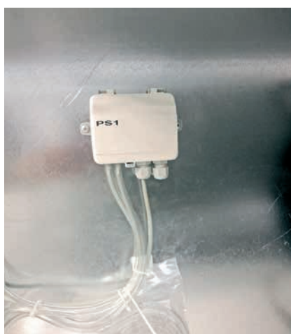
Figure 50: Pressure sensors unit with two differential pressure sensors. In CompAir it is used for measuring pressure in duct and also for measuring air flow of inlet and outlet fans. Communication with controller is via EXOline communication.
