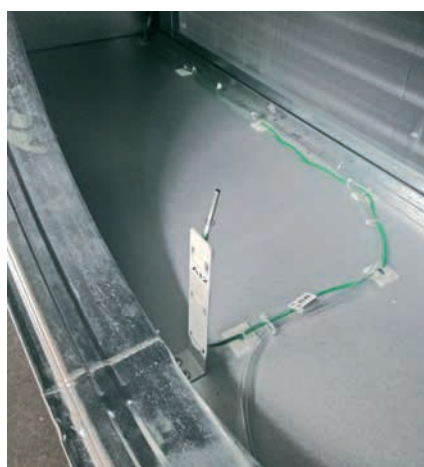
Figure 52: Temperature sensor for inlet air temperature. It has to be connected in the connection box located behind supply fan (green connector – see Figure 53).
