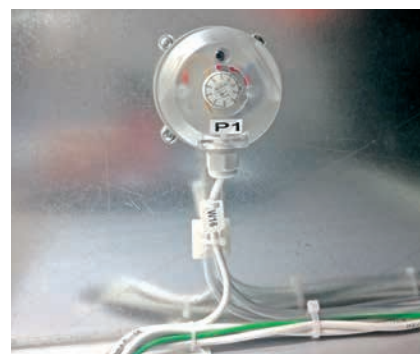
Figure 50: Differential pressure switch for fresh air or extract air filters.
