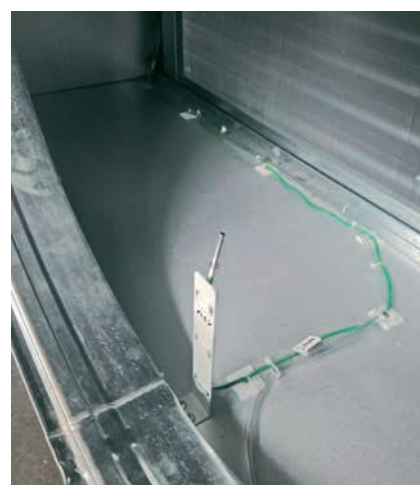
Figure 53: Temperature sensor for inlet air temperature. It has to be connected in the connection box located behind supply fan (green connector – see Figure 54
